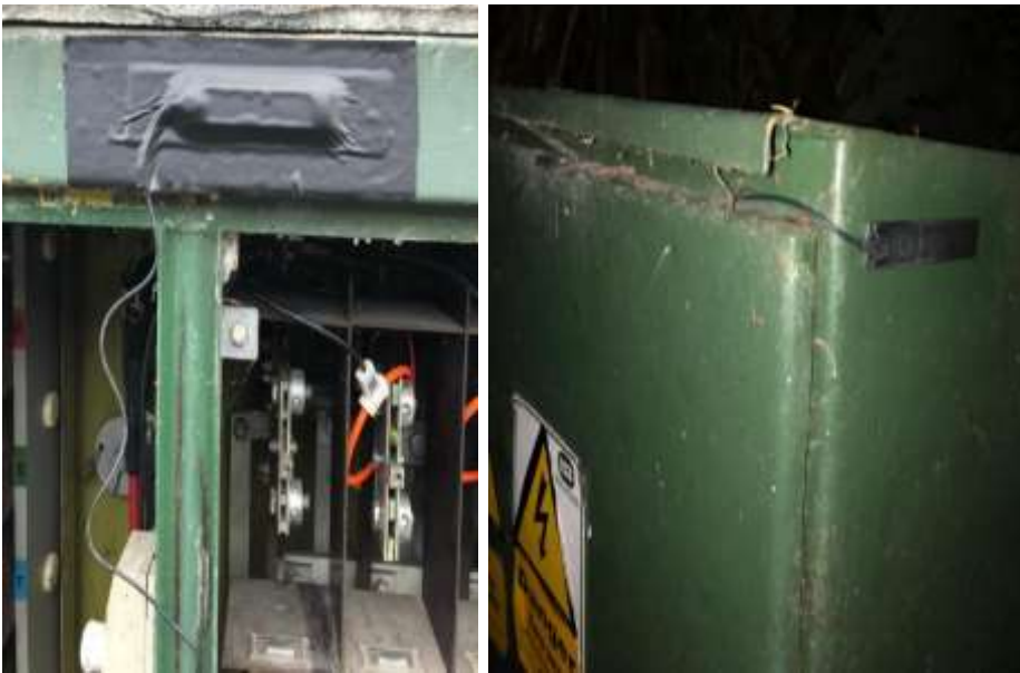
FIGURE 16: EXTERNAL PATCH ANTENNA PROTOTYPE
