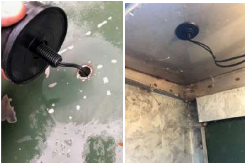
FIGURE 18: INSTALLING A PUK ANTENNA
