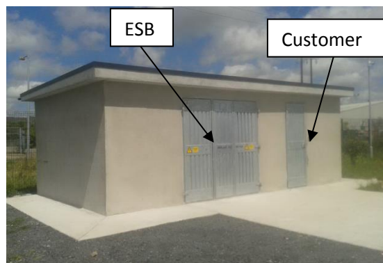
Fig. 2: Freestanding MV substation adjoining a customer's switchroom.
