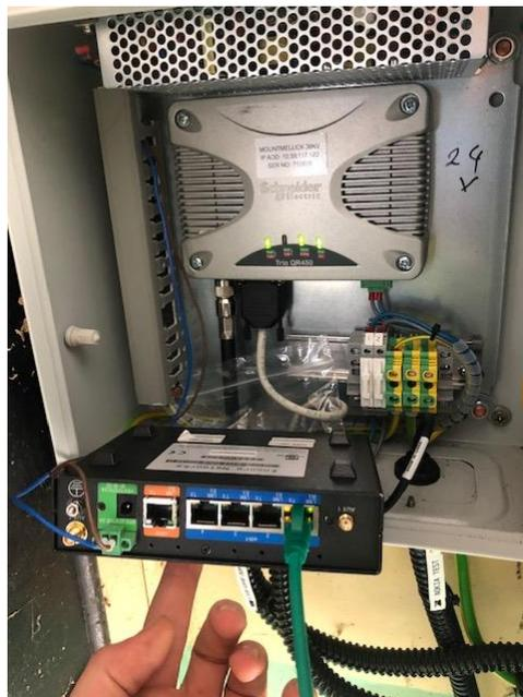
Figure 3: Vendor equipment field trial testing Portlaoise
