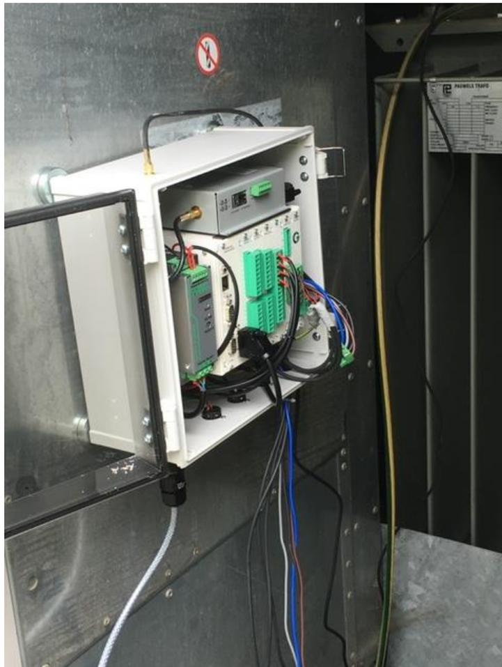
Figure 1: LV monitoring equipment connected to wireless transceiver.
