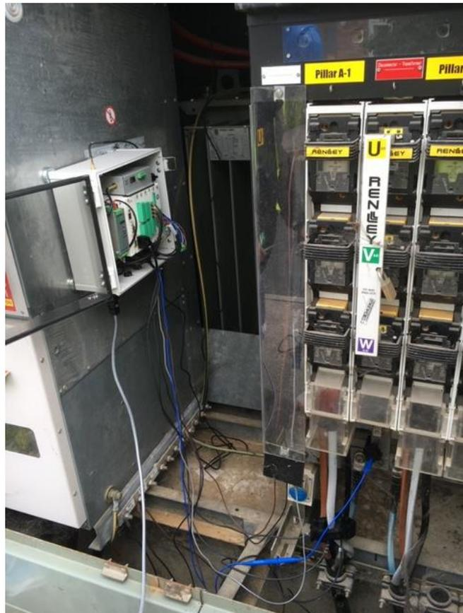
Figure 2: Wireless LV Monitoring device connected to a live substation.
