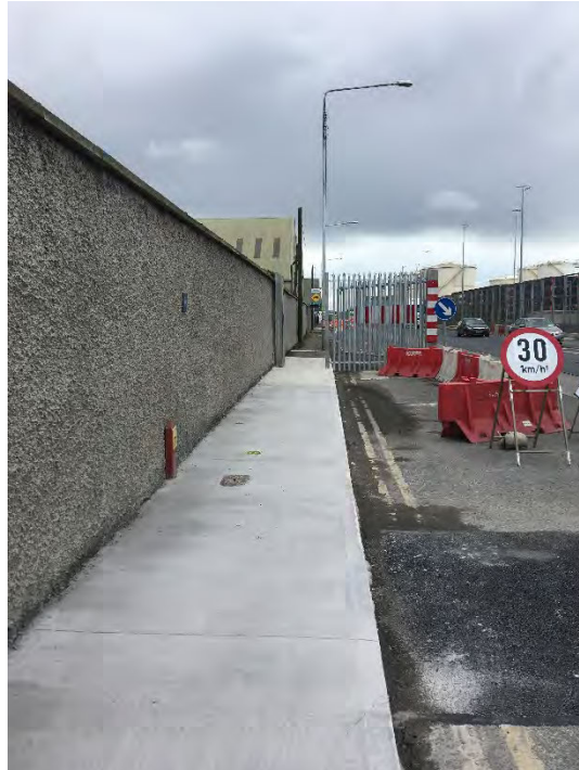
Photograph 1 – Leak location looking west
