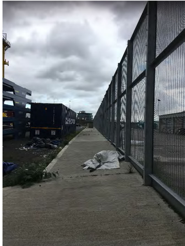
Photograph 3 – Cable route north to Tolka Quay Road
