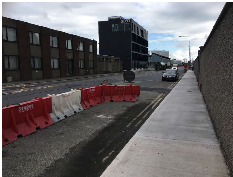
Photograph 2 – Leak location looking east
