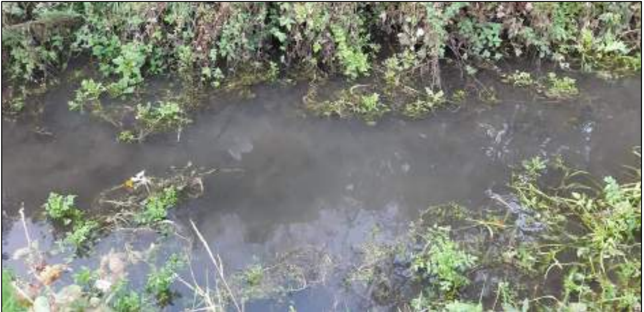
Photo 6: Image of nearest drainage channel, north of leak point, showing the poor water quality and stagnant water observed.
