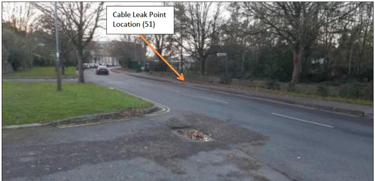
Photo 2: Looking west from entrance to nearby office complex; view of Monaghan Road. Note that cable leak point is located under pathway.
