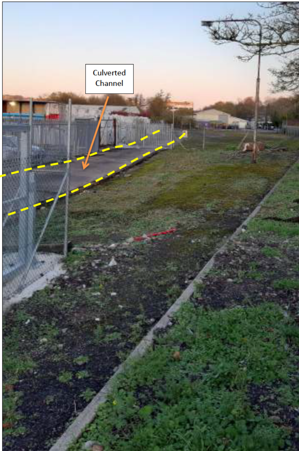
Photo 8: View, looking east, of a commercial property c.280m west of leak point, showing the concrete, culverted route of the drainage channel (flowing east). Note the Greenstar recycling facility in the far background.
