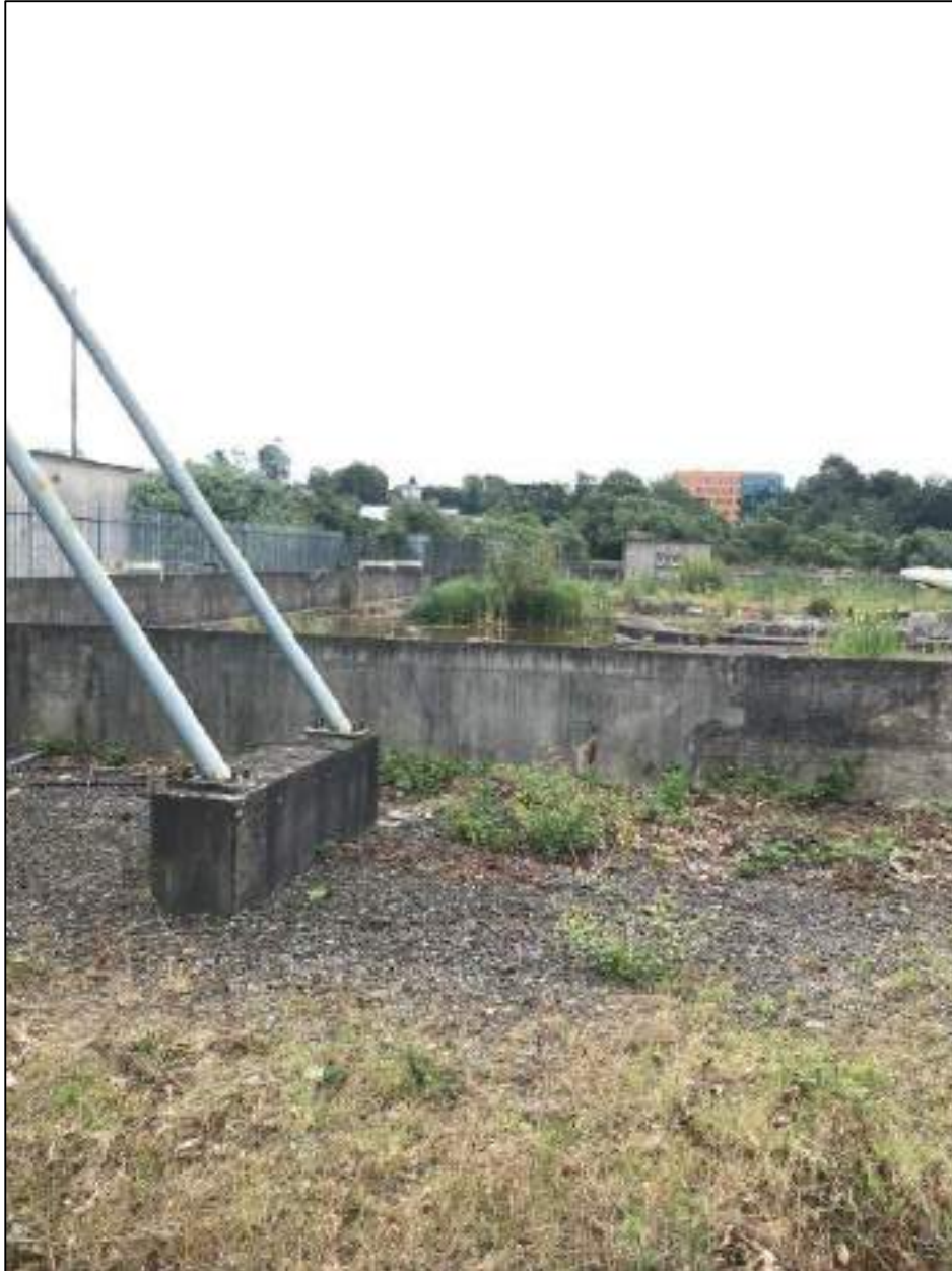
Photo 10: View from north side of decommissioned fuel storage depot on southern side of Centre Park Road. Note that the tree line in the background marks the boundary of the fuel facility and the location of the drainage channel. The 110kV cable runs along the left hand side of this image, towards the leak point.
