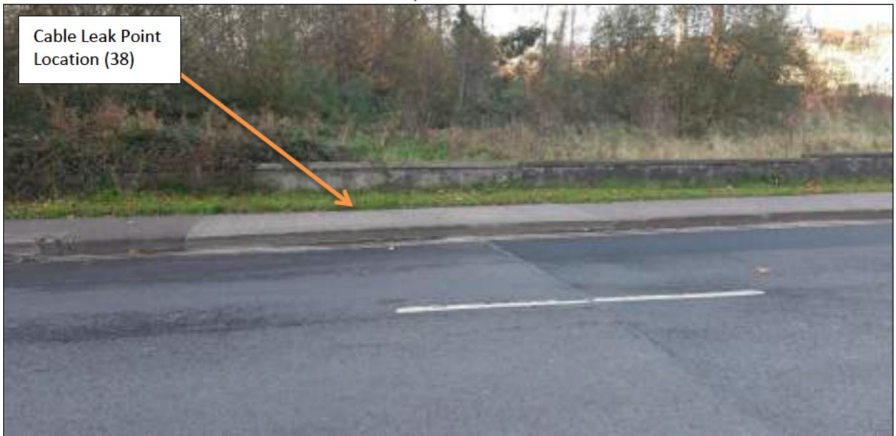
Photo 3: View north from Monaghan Road looking into section of concrete pathway that is associated with the leak point 38.
