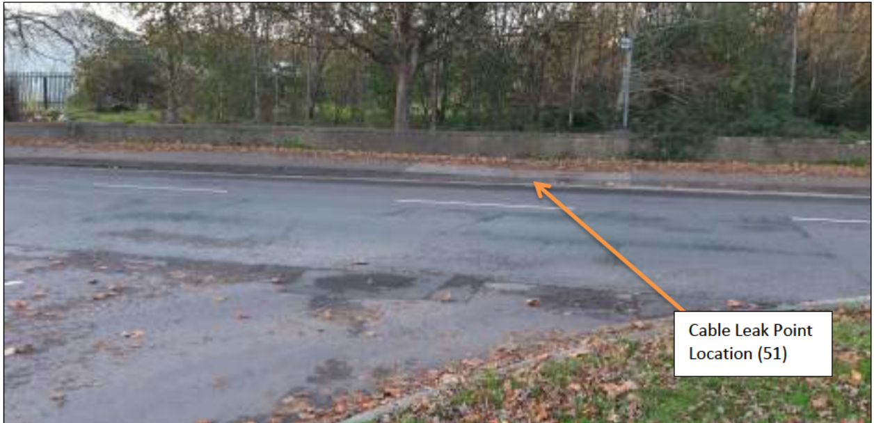
Photo 1: View north from Monaghan Road looking into section of concrete pathway that is associated with the leak point 51. Cable progresses north and west from this point. Note green area in background extends for c.50m to north where drainage channel is located.
