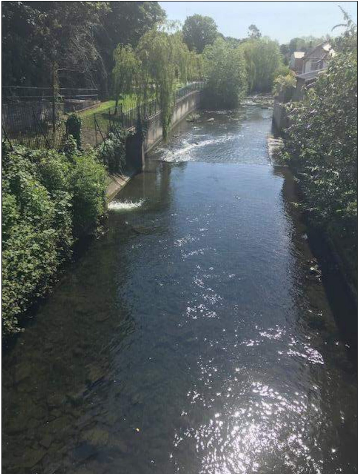
Photo 8: Tolka River approx. 890m south west of leak point
