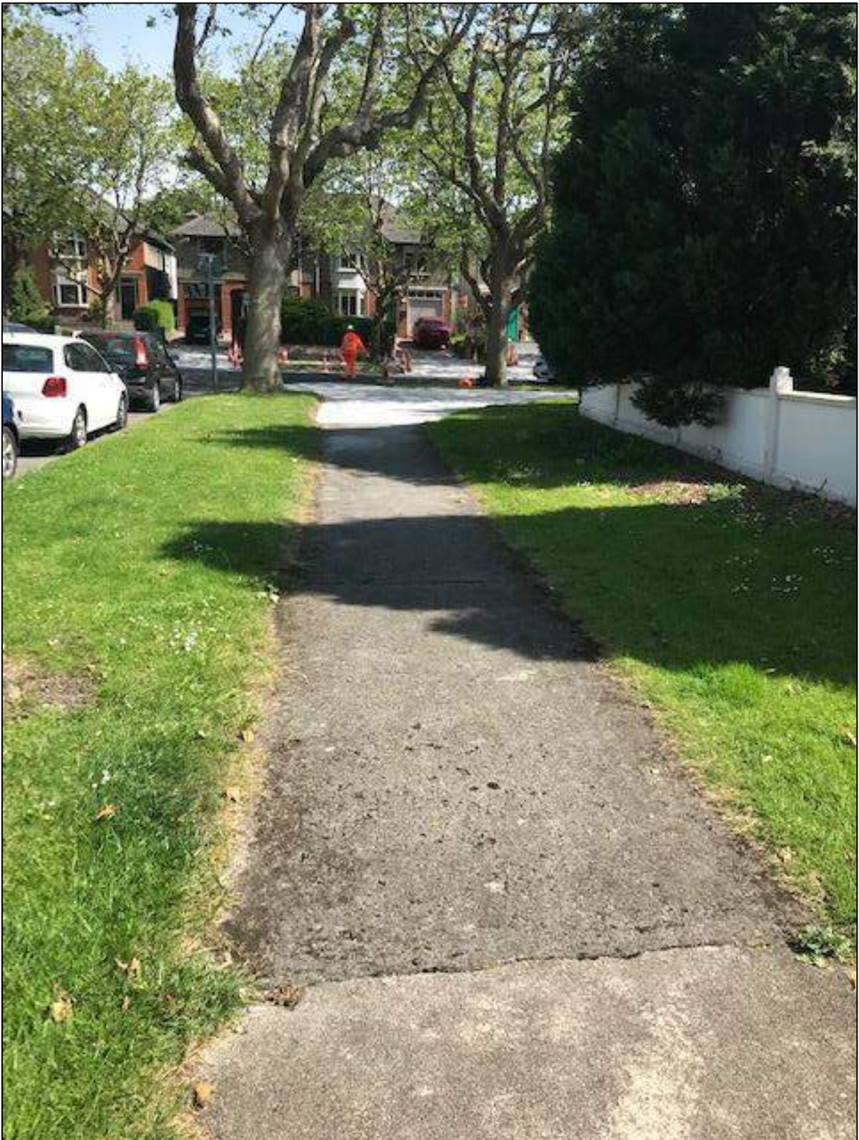
Photo 3: Area downgradient of leak point
