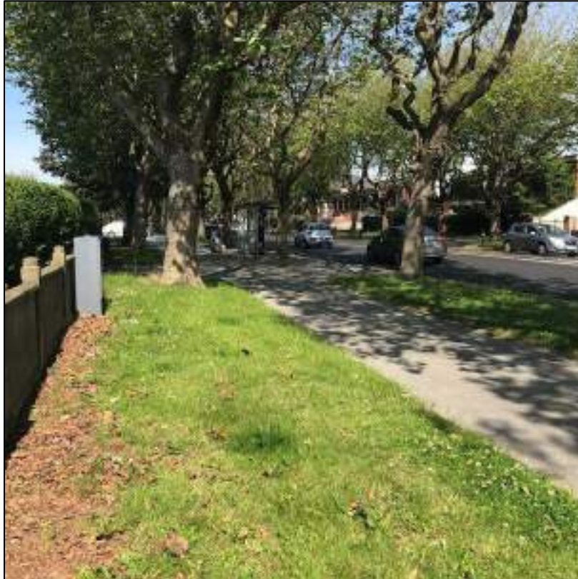
Photo 6: ESB Kiosk approx. 135m east of leak point.
