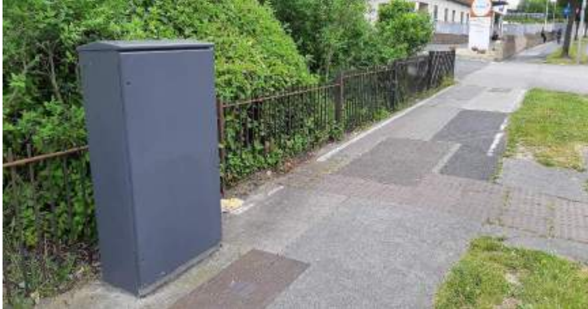
Photo 9: Area just south of the know leak site. See entrance to nursing home on LHS followed by repaired wall. Area of gravel around sign inside perimeter.
