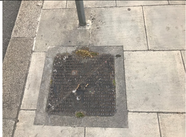
20-02 – Manhole present at Site on Burgh Quay.
