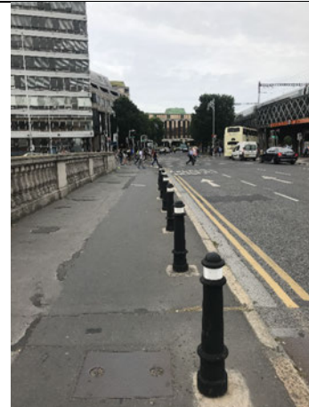
20-11 – Tarmac patching and resurfacing noted in footpath along Butt Bridge.
