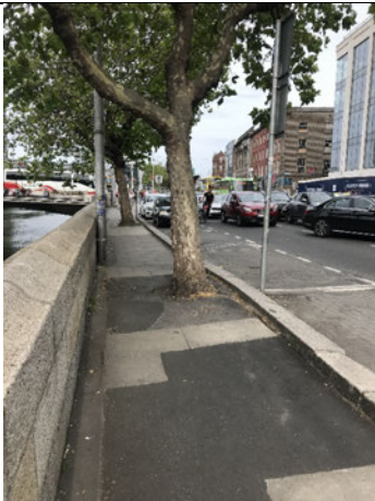
20-03 – Immature trees noted along the Burgh Quay footpath, however some more mature trees were noted between O'Connell bridge and Rosie Hackett Bridge. Potential for developed and mature root systems interacting with underlying services.
