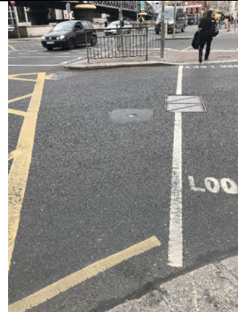
20-09 – Telecom and others manhole covers north of site at Beresford Place and Eden Quay.
