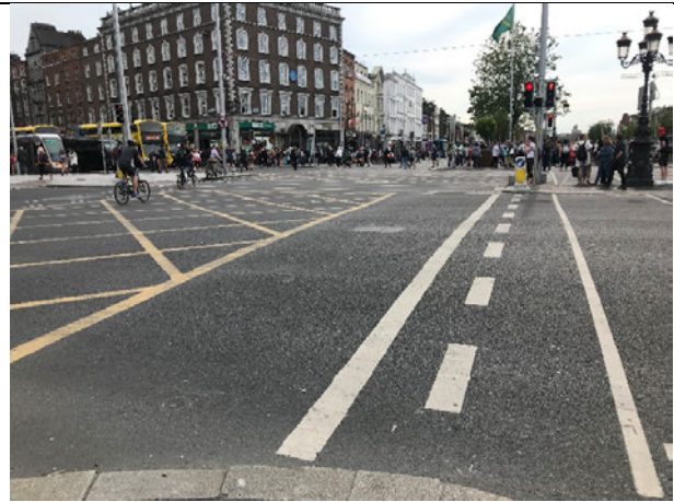
20-04 – Going west along the cable length; towards O'Connell bridge and Aston Quay the road surfaces appeared in good condition.
