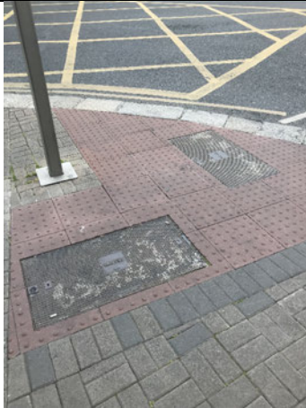
20-08 – Telecom and others manhole covers north of site at Beresford Place and Eden Quay.
