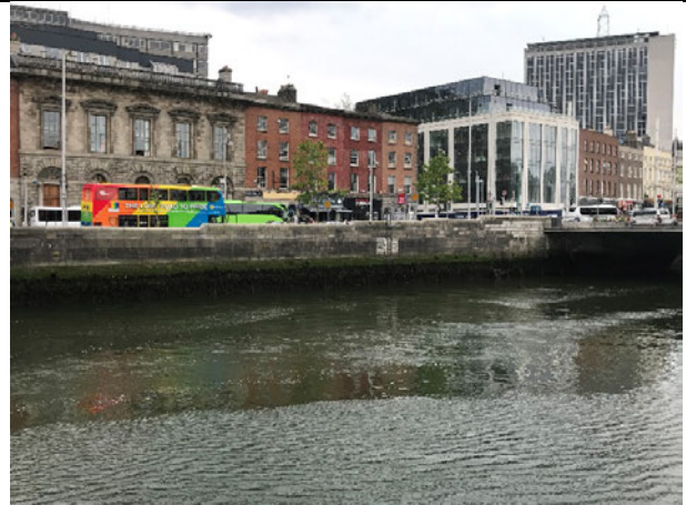
20-05 – Algae, seaweed, dirt and debris noted on quay wall (observed from opposite side of the river and Rosie Hackett Bridge). From a distance, no obvious inconsistent appearance on quay wall.
