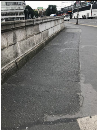
20-10 – Tarmac patching and resurfacing noted in footpath along Butt Bridge.
