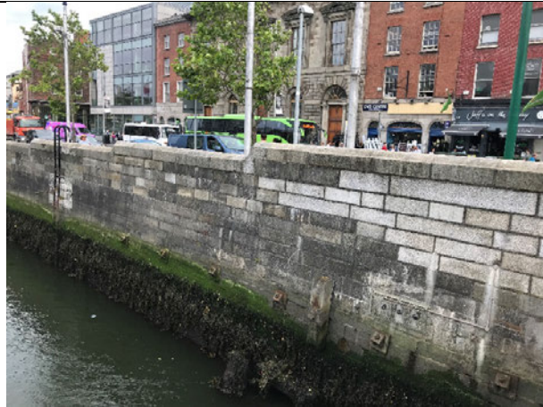
21-00 – Algae, seaweed, dirt and debris noted on quay wall (observed from opposite side of the river and Rosie Hackett Bridge). From a distance, no obvious inconsistent appearance on quay wall.
