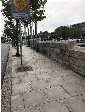
20-01 – Footpath appearing in good condition at the Site.
