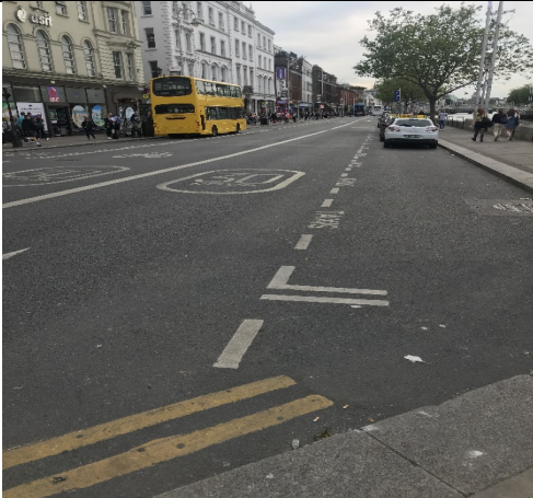
20-04 – Going west along the cable length; towards O’Connell bridge and Aston Quay the road surfaces appeared in good condition.
