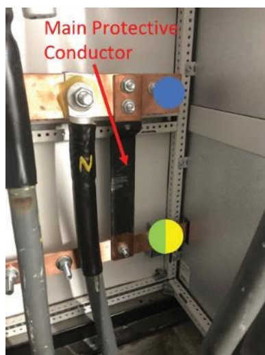
Figure 7: Example of TN-C-S in a commercial installation
