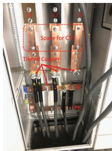
Figure 9: Single Commercial installation >200 kVA
