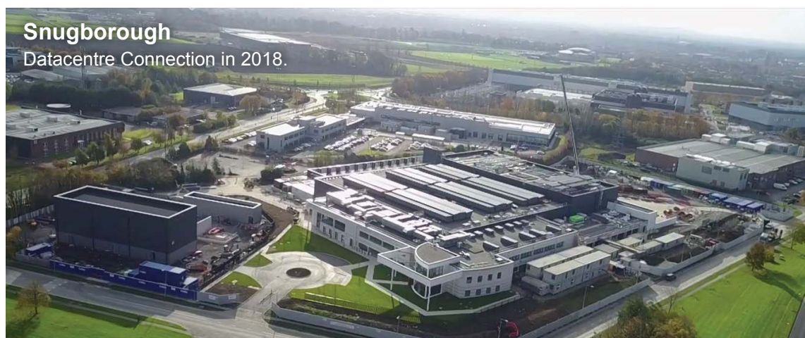
Snugborough 110 kV GIS in foreground located adjacent to datacentre
