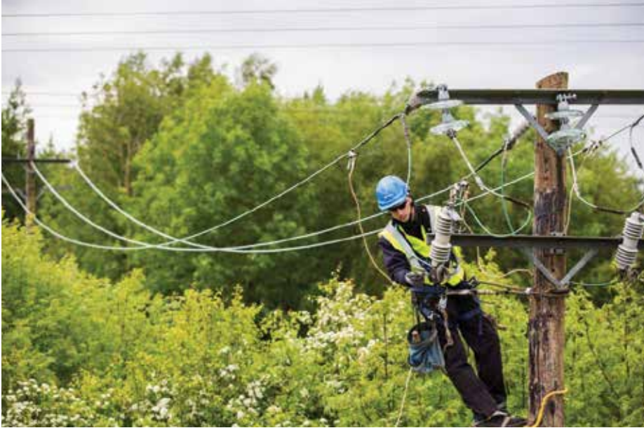
Network technician repairing fallen wires after a storm.
