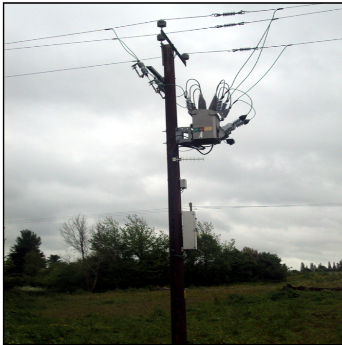
Figure 1. MV Pole Mounted Recloser
