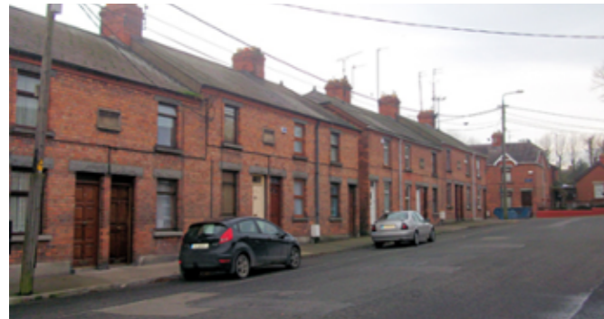
Figure 4: LV cables - black wiring on house frontage
