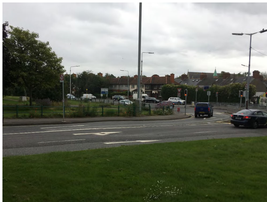
Photograph 2 – Looking towards leak location from north-east
