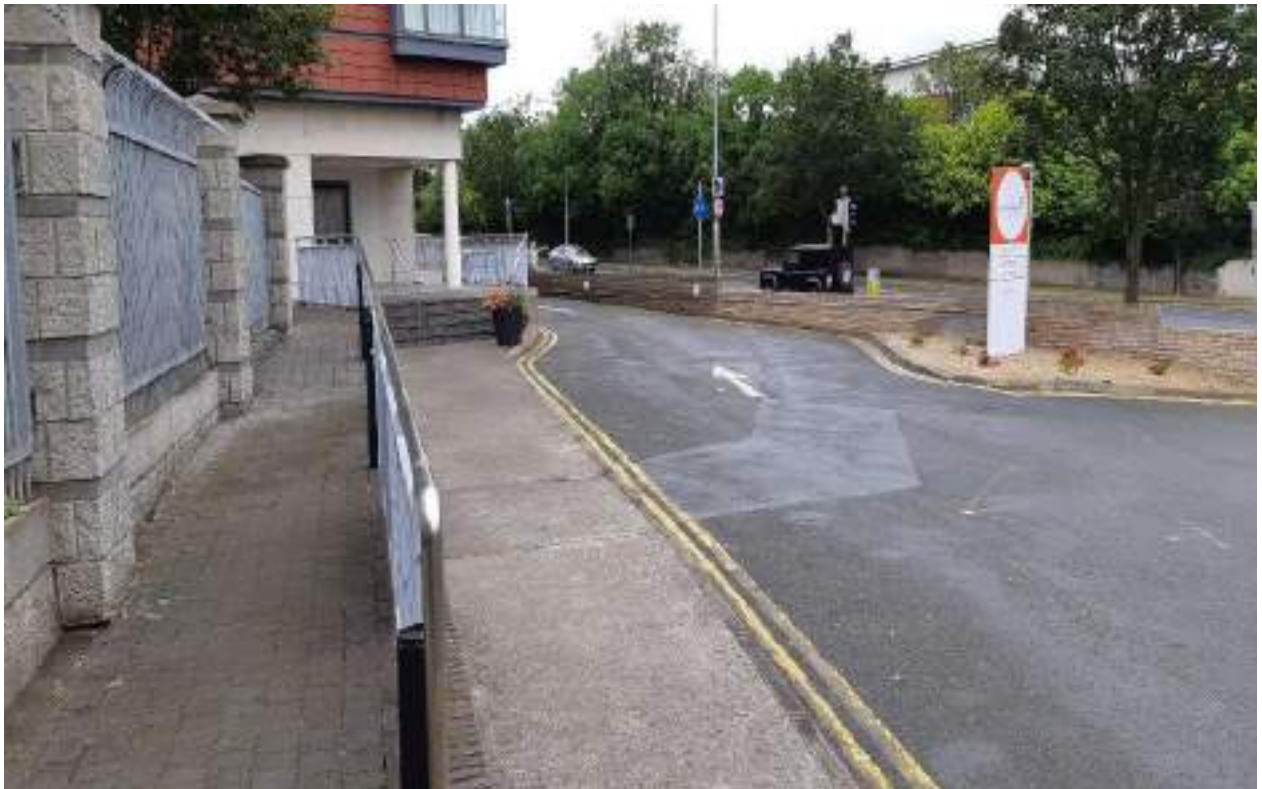
Photo 4: Outline of trench leading from ESB substation across set-down route for nursing home
