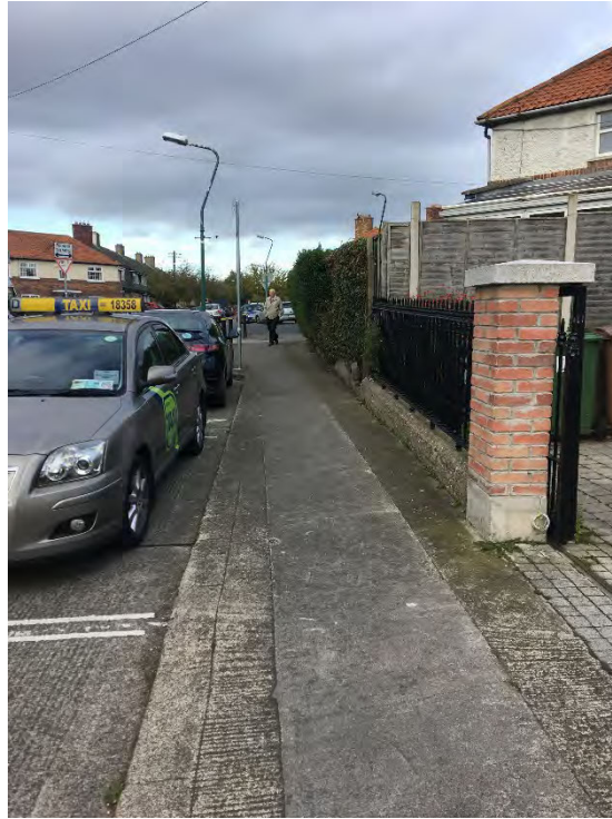
Photograph 1 – Leak location looking north-west
