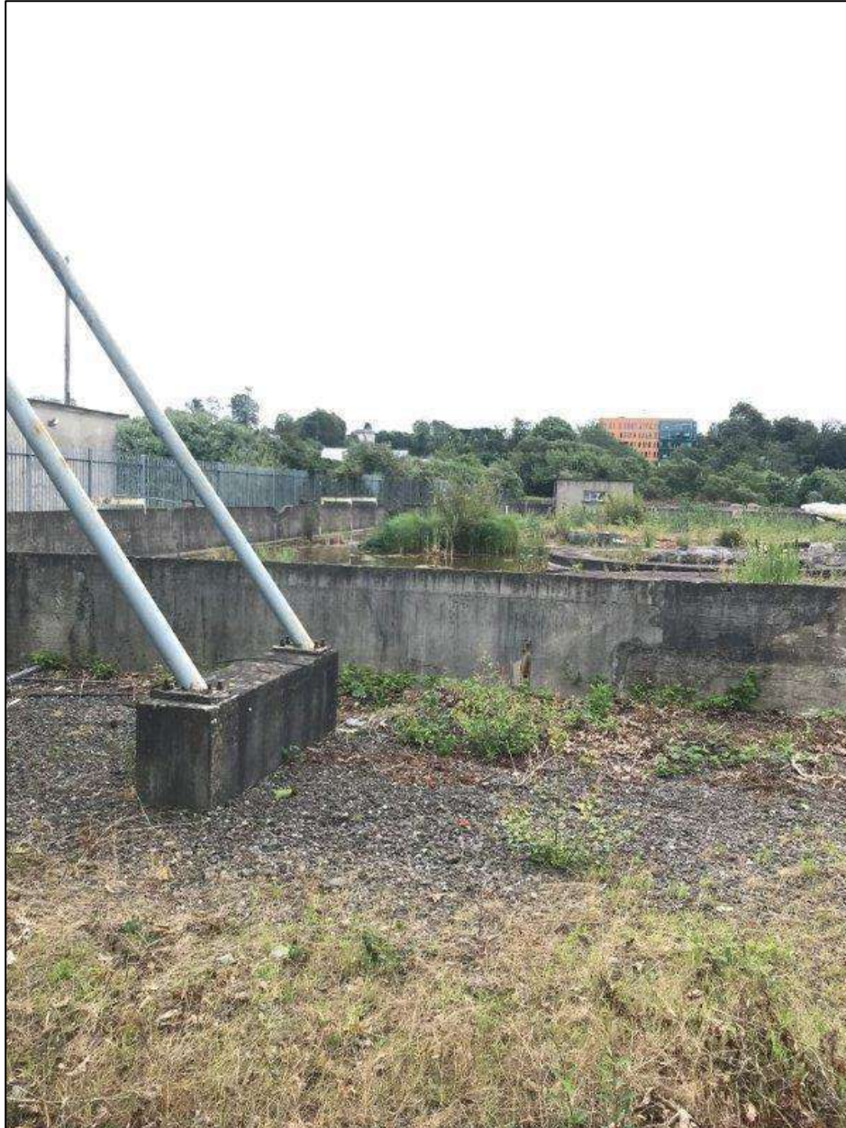
Photo 10: View from north side of decommissioned fuel storage depot on southern side of Centre Park Road. Note that the tree line in the background marks the boundary of the fuel facility and the location of the drainage channel. The 110kV cable runs along the left hand side of this image, towards the leak point.
