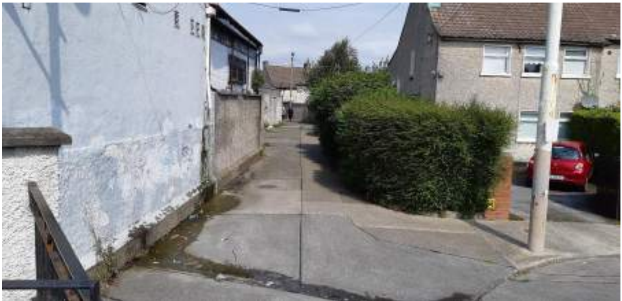
Photo 17: Laneway that connects two areas of O'Rourke Park. Cabling is understood to run along this laneway.
