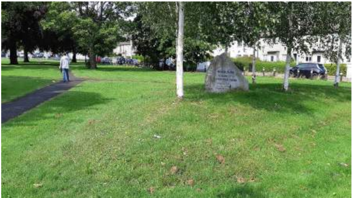
Photo 15: Cables traverse Wood Park in southwest direction to RHS of central path. No evidence on surface of leaks.
