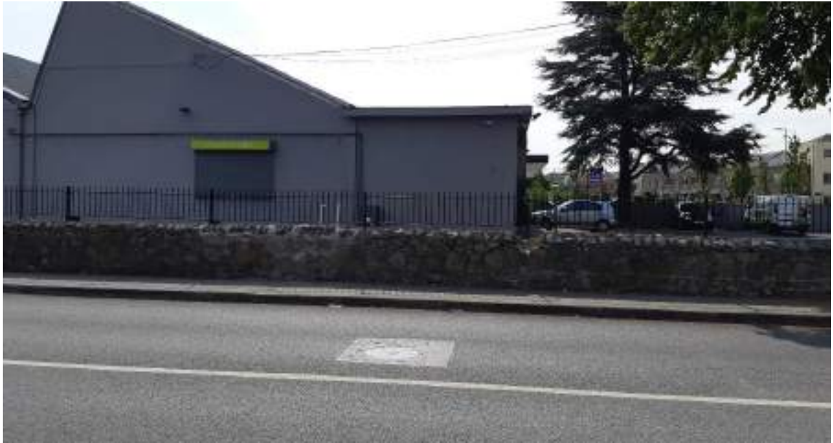
Photo 3: View of repaired wall and Davies Showroom from Sallynoggin Road. Leak site is far side of repaired wall.
