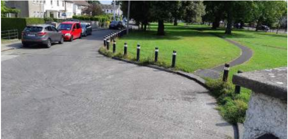
Photo16: At southwest corner of Wood Park, cables cross parking circle at end of O'Rourke Park residential estate. Cables veer to right and travel up narrow laneway which connects to further area of estate
