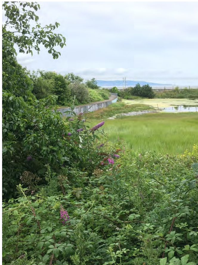
Photograph 2 – Looking east from leak location
