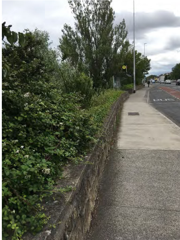
Photograph 5 – View south along Rock Road
