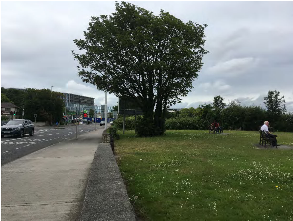
Photograph 1 – Leak location adjacent to Rock Road
