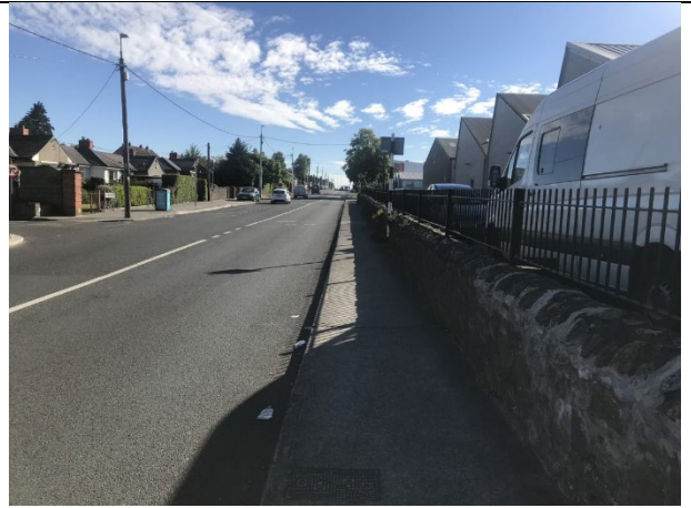
14-04 – Road surfacing in generally good condition on Sallynoggin Road.
