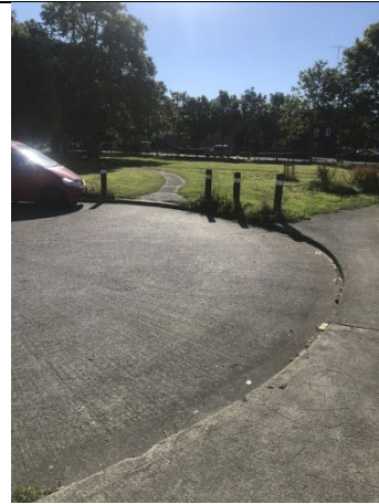
14-08 – No evidence of surface works, surface staining or dieback to the southwest of the Site at O'Rourke Park.
