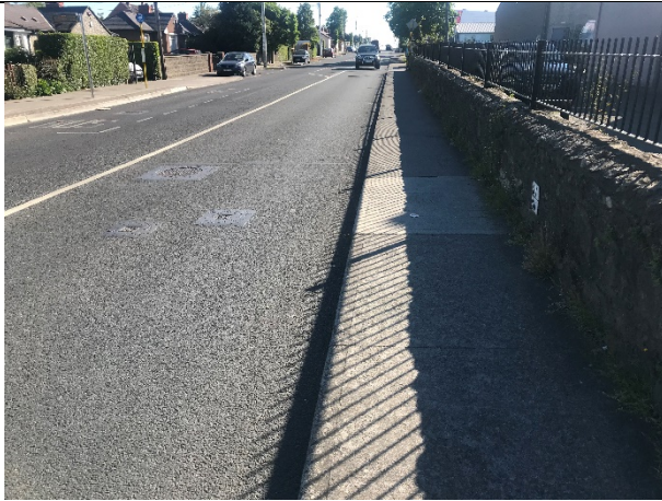
14-03 – Conduit covers on Sallynoggin Road adjacent to indicative leak location.
