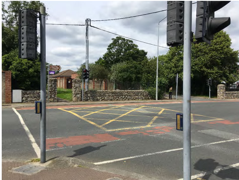
Photograph 1 – Leak location; west side of Brewery Road
