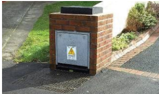
← Example of Minipillar installed between two driveways.
