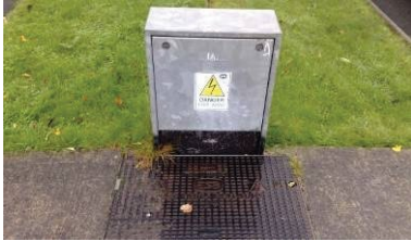
← Example; Finished Minipillar in open plan site
