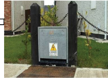
Example; Finished Minipillar in open plan site □
